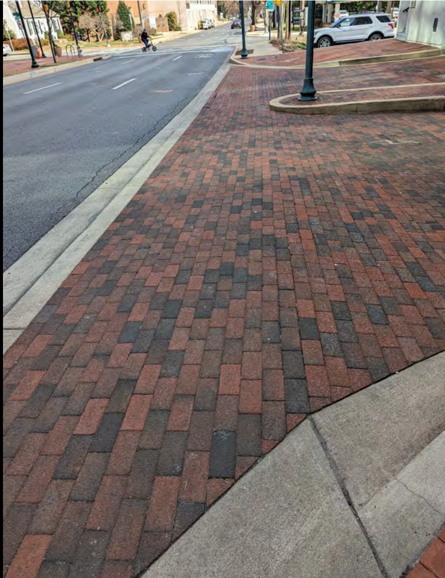
Montgomery Ave. Driveway curbs impede free flow and force pedestrians and wheelchairs close to the street
