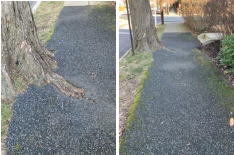
Flexi pave installed in Georgetown
