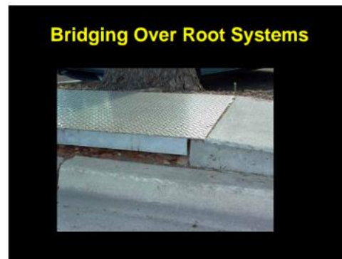
Sidewalk "bridges", leaving air space for roots to survive and thrive
