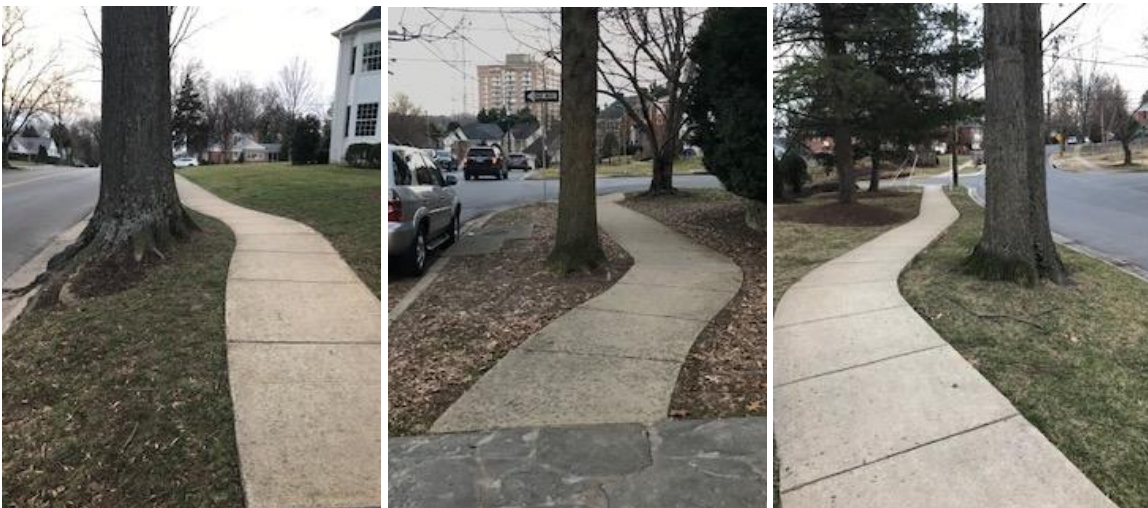
Curved cement sidewalk working around trees. Ridgefield Road in Westbard neighborhood, Bethesda
