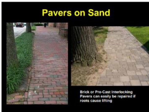
Alternative porous pavement materials
