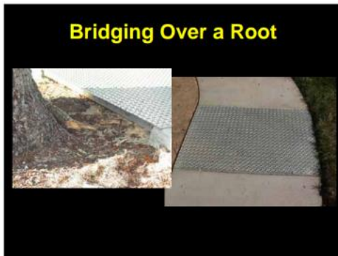
Sidewalk "bridges", leaving air space for roots to survive and thrive
