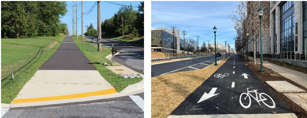
Figure 9: Photos of Sidepath (left side) and Two-Way Separated Bike Lanes (right side)
