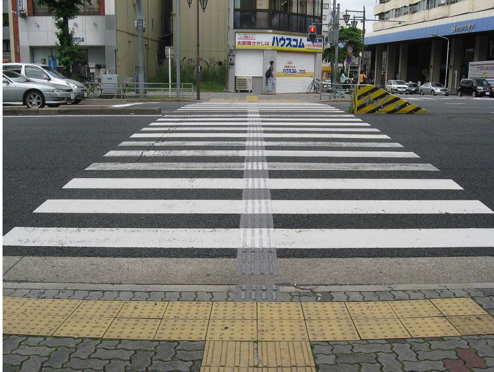
A tactile crosswalk in the center of the painted crosswalk in Japan. Courtesy: Wikimedia
