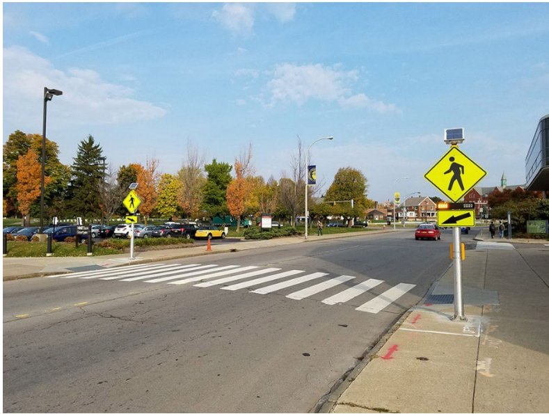
Figure 6 Example of Rectangular Rapid Flashing Beacon (RRFB)
