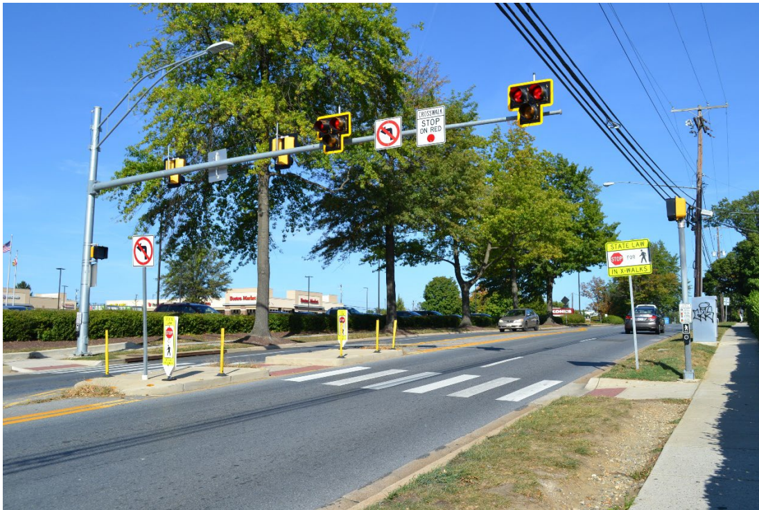
Figure 4 Pedestrian Hybrid Beacon - Aspen Hill Road
