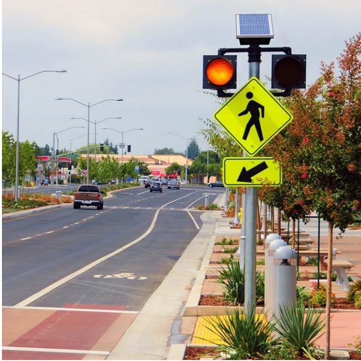
Figure 5 Example of Circular Flashing Beacon
