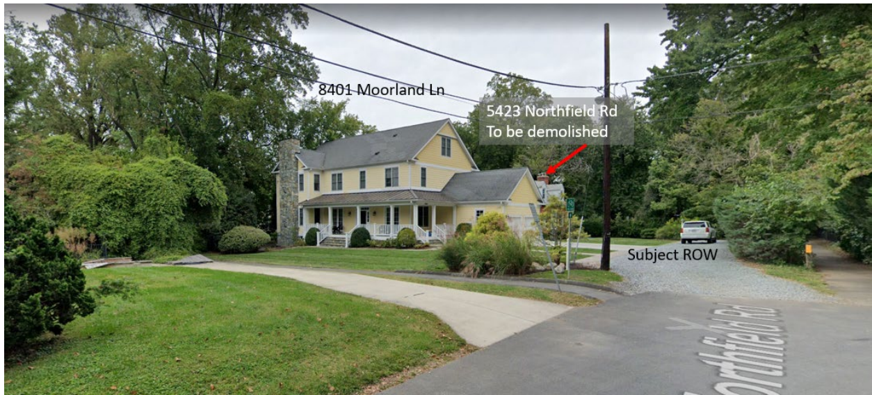
Figure 3 – View of Subject Abandonment (Northfield Road looking east)
