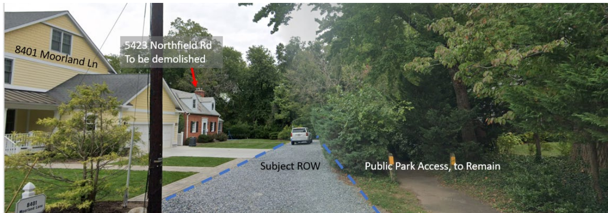
Figure 4 – View of Subject Abandonment, closer view (Northfield Road looking east)
