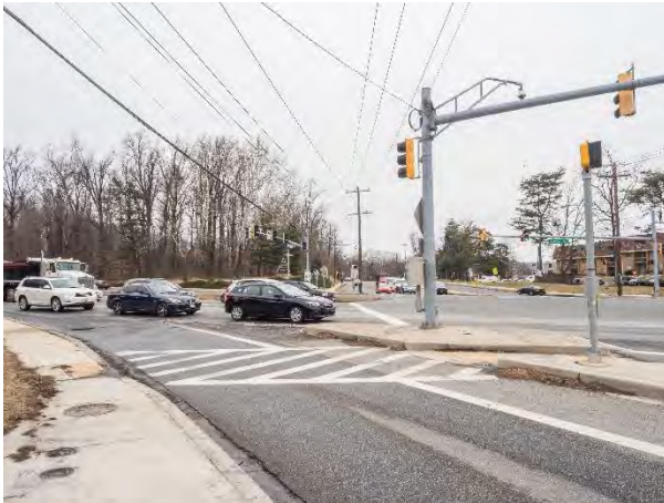
A channelized right turn lane with porkchop island at Bel Pre Road and Georgia Avenue
