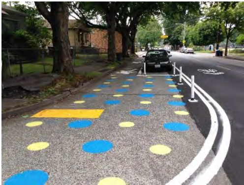
A painted pedestrian pathway in the street is separated from traffic by parked cars, temporary concrete curbs, and white flex posts. Photo Credit: Dongho Chang
