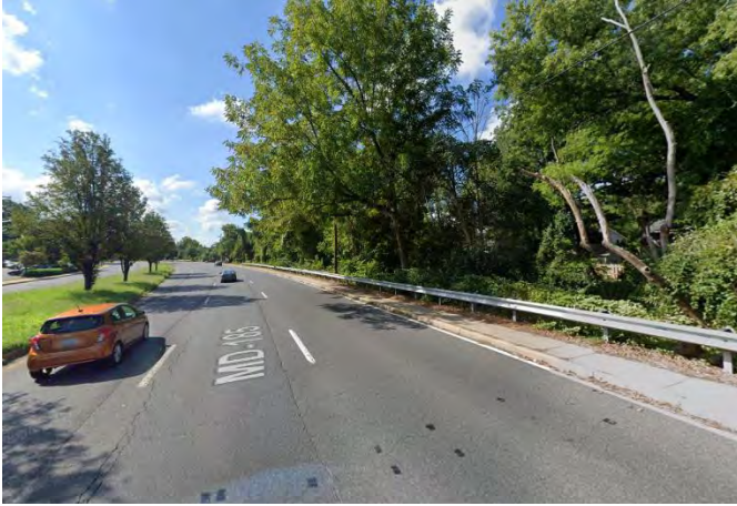
Guardrail behind sidewalk along Connecticut Avenue in Aspen Hill. Photo Credit: Google Maps
