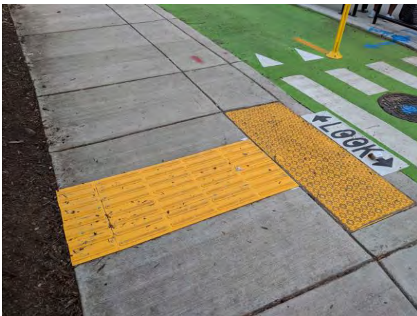
Example of a TWSI used in Montgomery County to direct people with vision disabilities to a floating bus stop.
