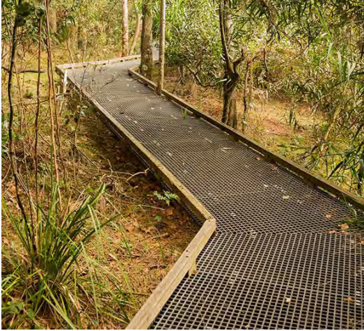
Metal boardwalk snakes through parkland. Photo Credit: Marco Specialty Steel
