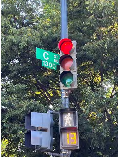
Pedestrians begin crossing the street while adjacent cars have a red signal.
