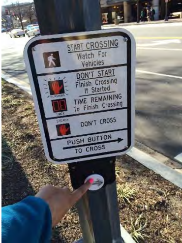
A pedestrian push button. Photo Credit: Montgomery County Government
