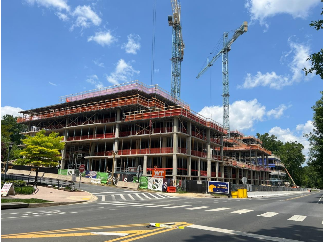
Figure 5 - Building 3 Construction (from Tuckerman Lane facing north)
