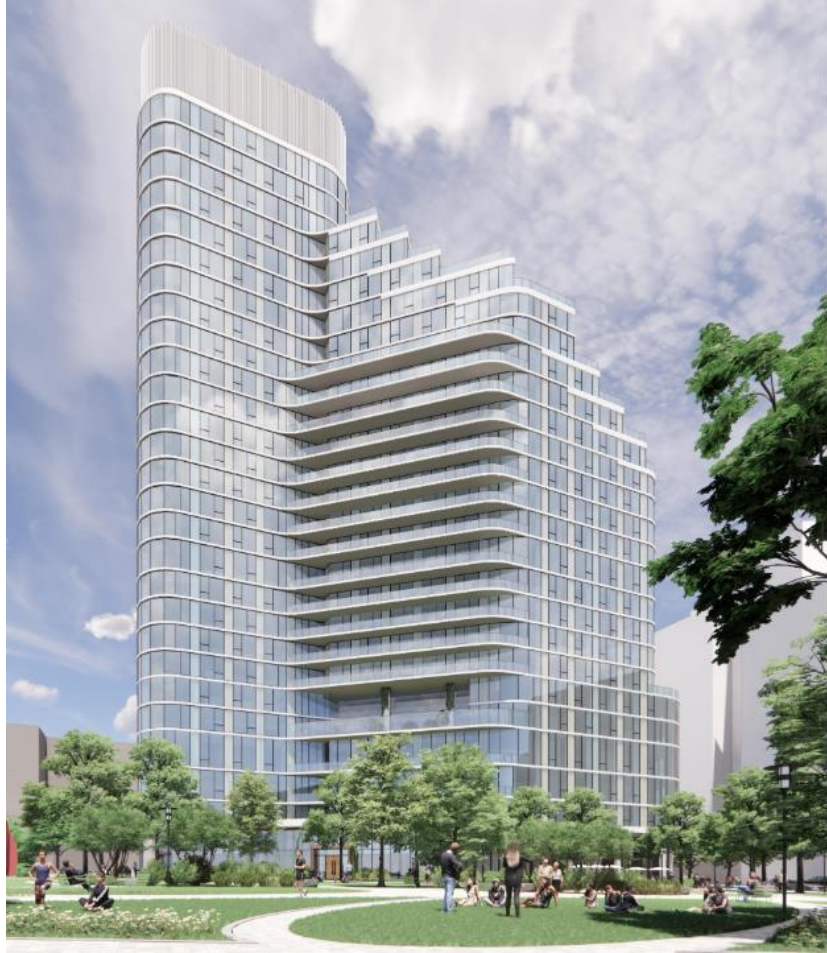
Figure 17 - Illustrative View of Building 5/The Reserve (from Central Park facing northeast)
