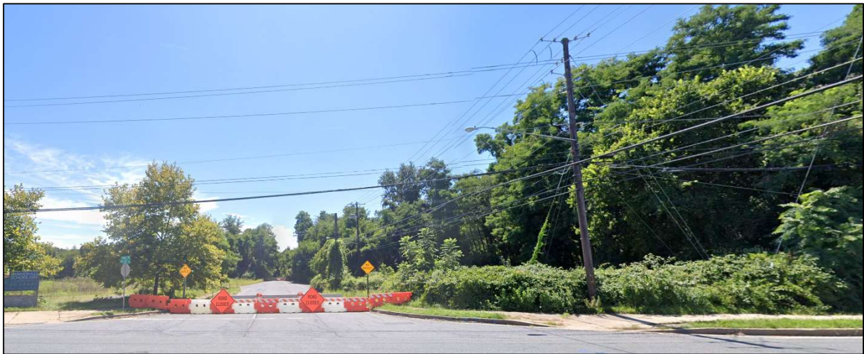
Figure 2 – Southward view of Liberty Mill Road, overhead power running south along west side of roadway
