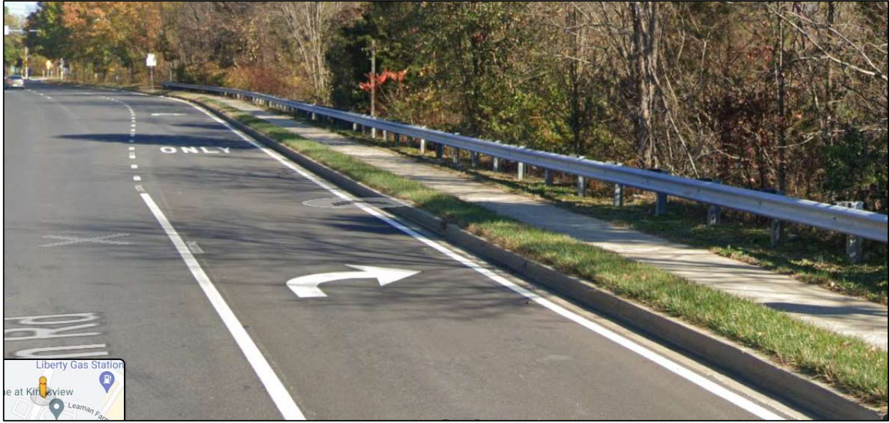
Figure 5 – Germantown Road Existing Sidewalk and Right Turn Lane
