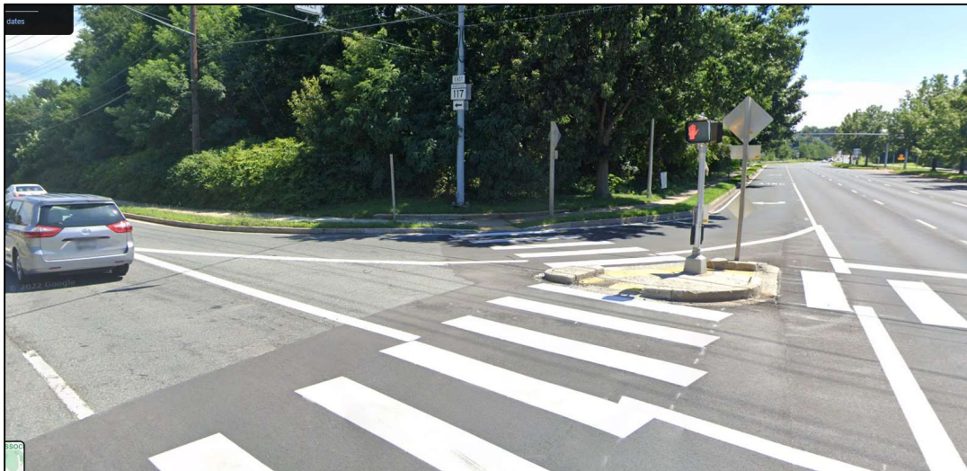
Figure 11 – Slip Lane to Be Removed at Germantown Road / Clopper Road Intersection
