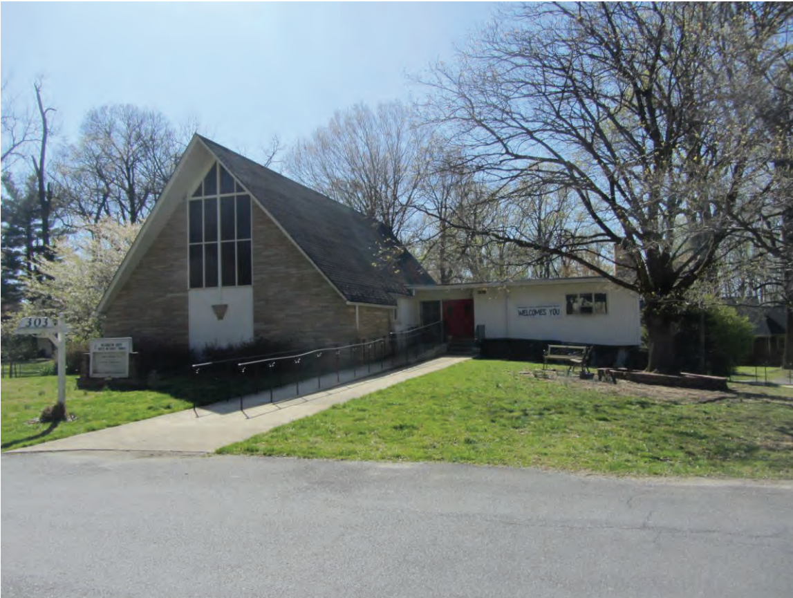
MD_MontgomeryCounty_WashingtonGroveHD_0039.tif 313 Chestnut Avenue (Washington Grove United Methodist Church), looking west
