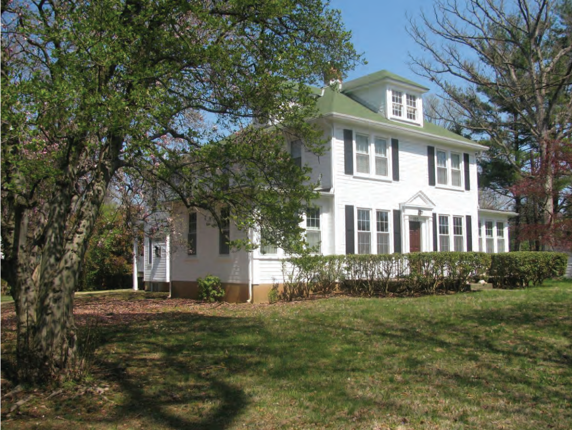
MD_MontgomeryCounty_WashingtonGroveHD_0029.tif 103 Brown Street, looking northeast
