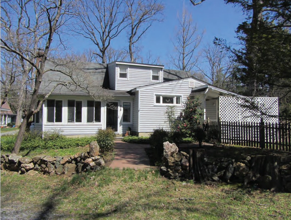
MD_MontgomeryCounty_WashingtonGroveHD_0021.tif 313 Grove Avenue, looking northeast
