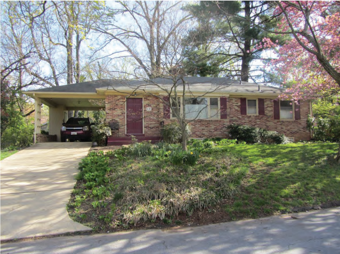
MD_MontgomeryCounty_WashingtonGroveHD_0036.tif 13 Center Street, looking north
