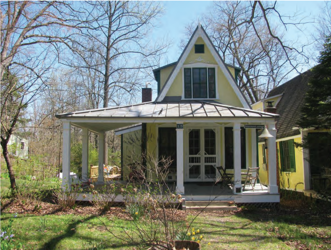
MD_MontgomeryCounty_WashingtonGroveHD_0019.tif 15 the Circle, looking east
