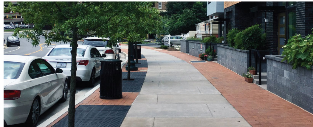
Example of streetscape in downtown Silver Spring that combines poured-in-place concrete areas with unit paver areas.
