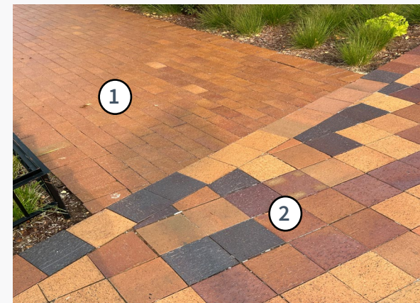
Example of Sidewalk Zone (1) and Buffer (2) paving material.
