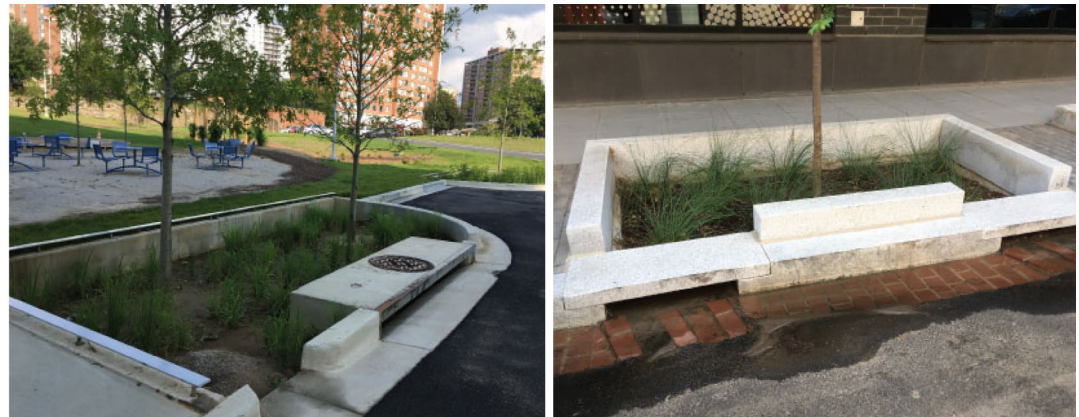
Examples of Infiltration Planters
