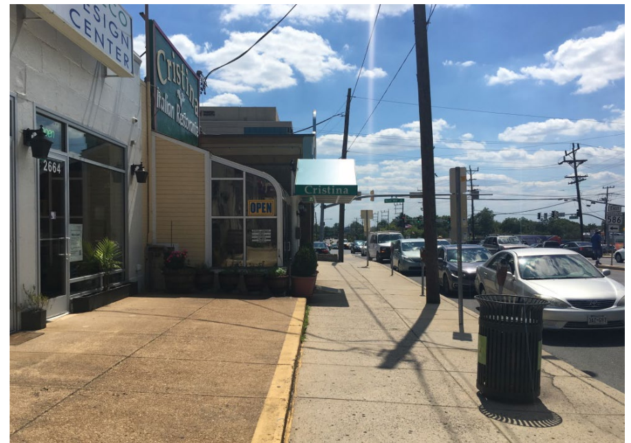
Examples of various existing sidewalk conditions in downtown Wheaton.
