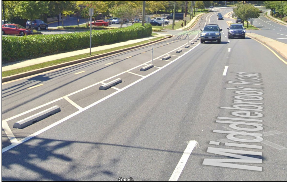
Figure 15 - Middlebrook Road Example Road Diet
