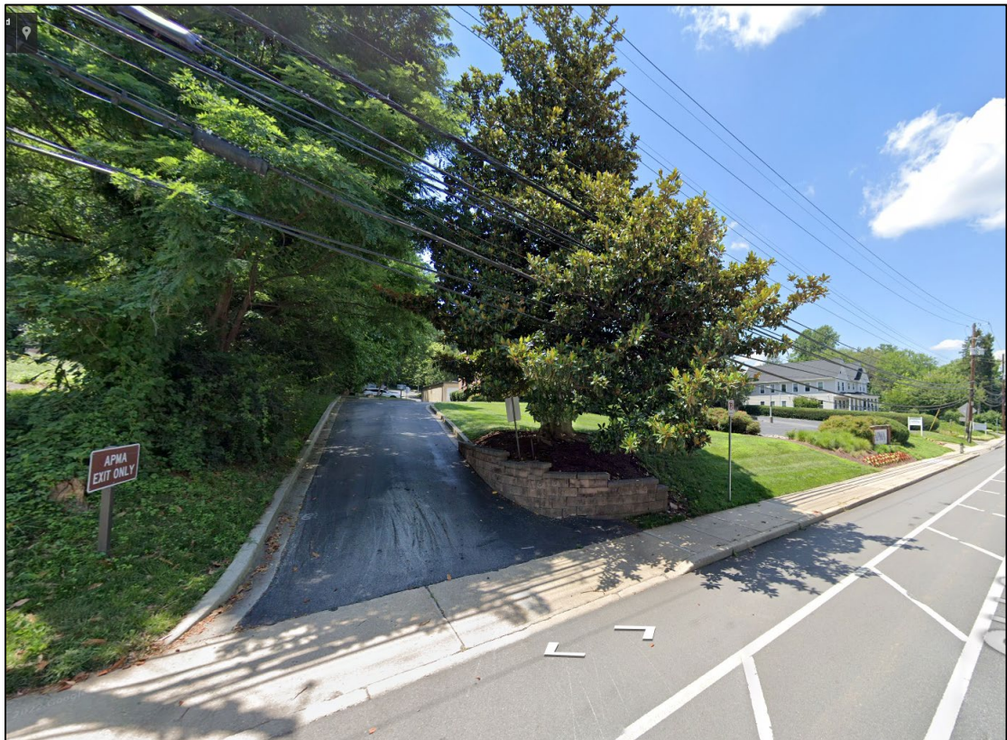
Figure 4: South End/Exit Driveway of Subject Property
