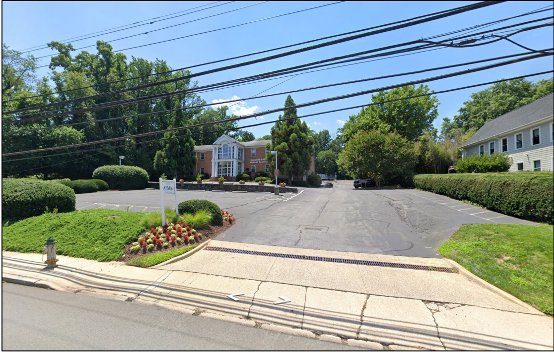
Figure 3: North Entrance of Subject Property
