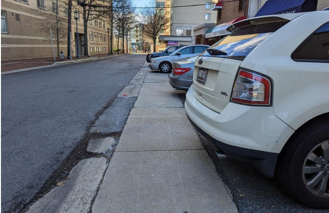
Figure 13 – Existing sidewalks on Miller Avenue
