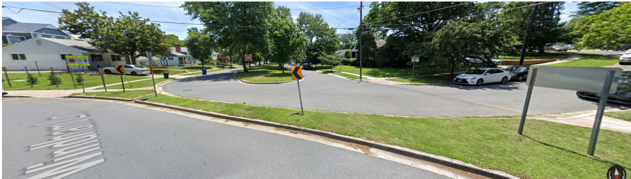
Image 5: Street view of the existing Douglas Avenue diagonal diversion.
