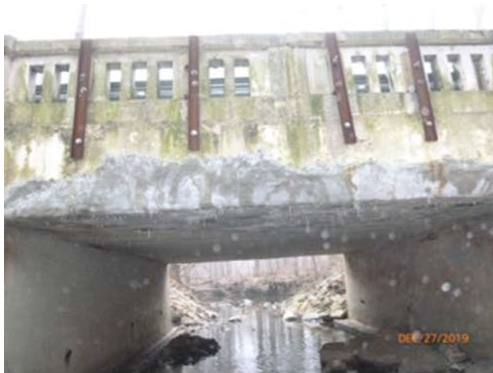
Delaminated Concrete
