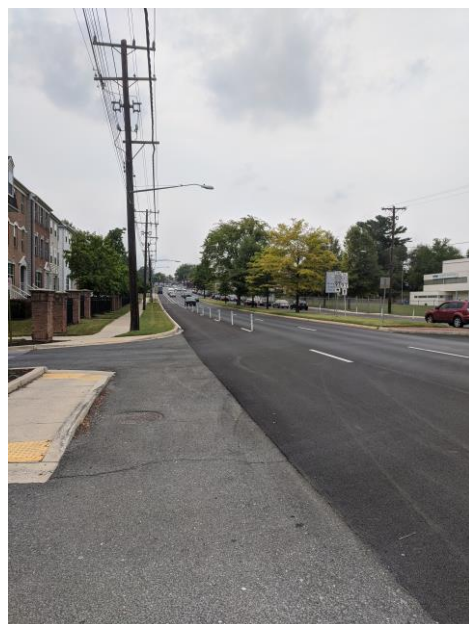
SHA Temporary Bikelane
