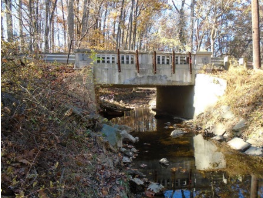
Figure 2: Existing Redland Road Bridge over Mill Creek
