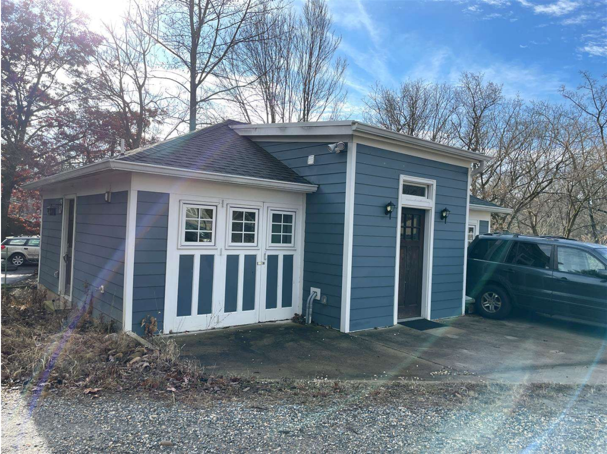
Figure 9: North (front) and east elevations of the former garage, view to southwest, Nancy LiPira, December 9, 2022.
