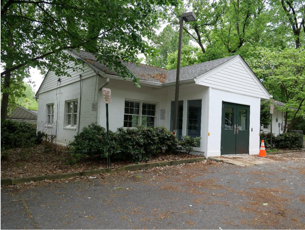
Figure 7: View of the northeast corner.
