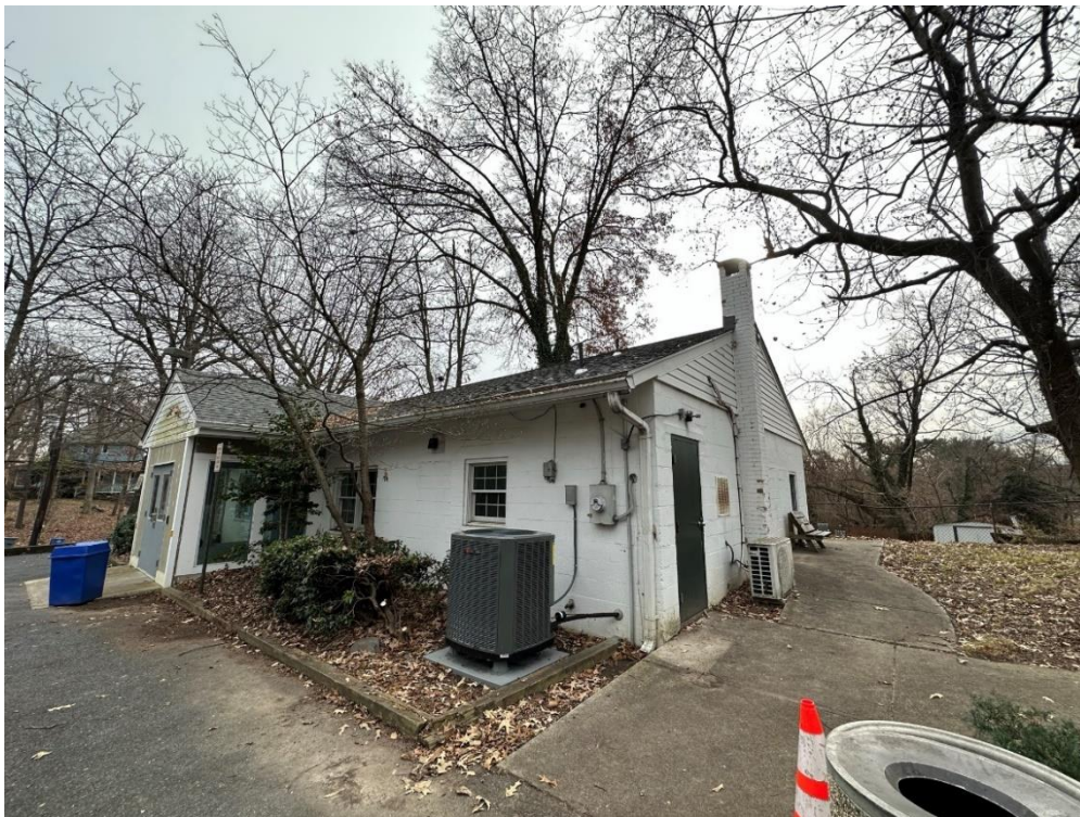
Figure 2: View of the northwest corner.
