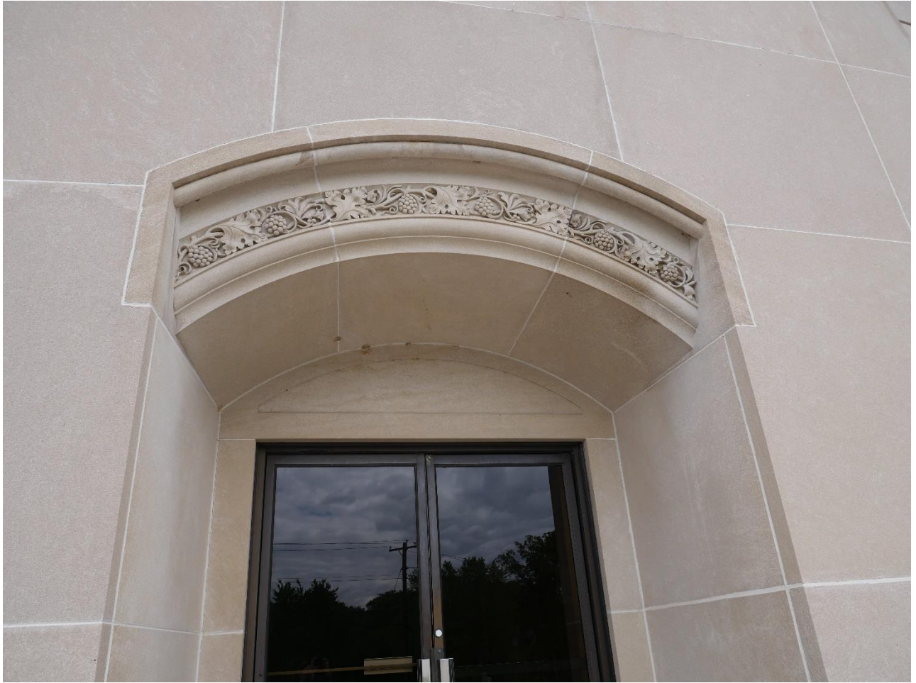
Figure 3: Detail of low-relief stonework in projecting entry bay. Source: Montgomery Planning.
