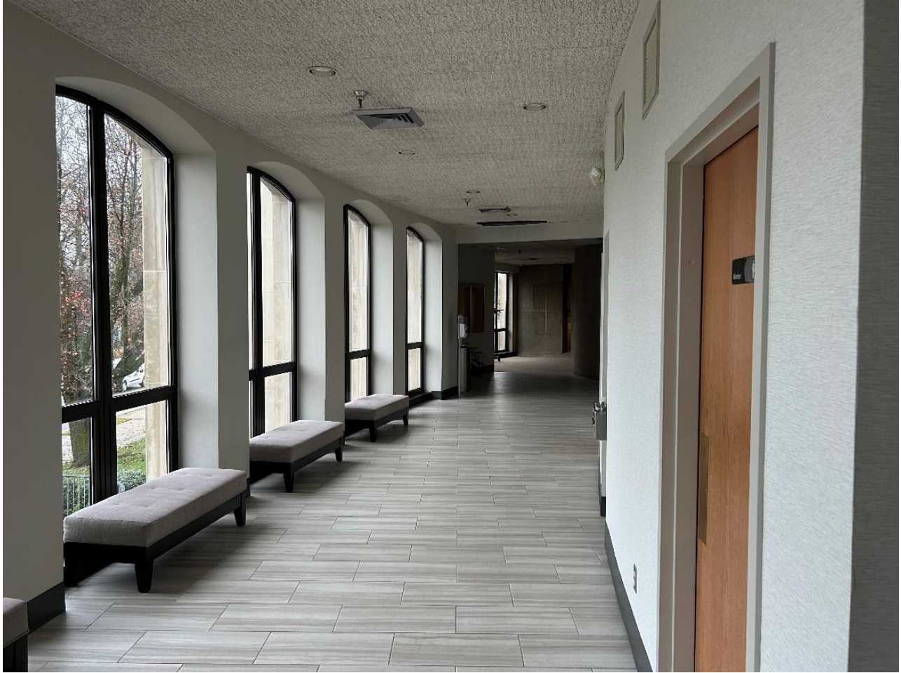
Figure 15: Interior of central pavilion of 1985 addition, looking northwest. Source: EHT Tracerries, Inc.
