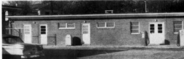
Personnel have not been forgotten; this part of the maintenance building houses separate shower and locker facilities for highway and sanitation divisions.
