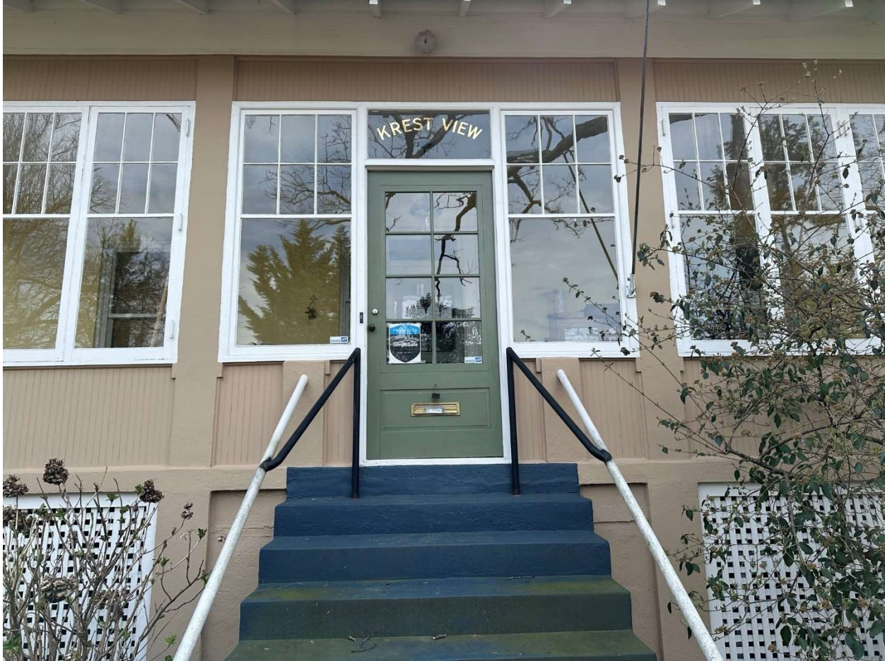
Figure 2: Detail of enclosed porch on front (north) elevation and transom window with “Krestview” name. Montgomery Planning, March 22, 2023.
