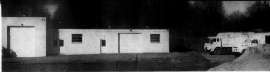
Three equipment repair bays (one is shown at left), a carpenter shop plus ample storage space provide the best in working conditions and facilities.
