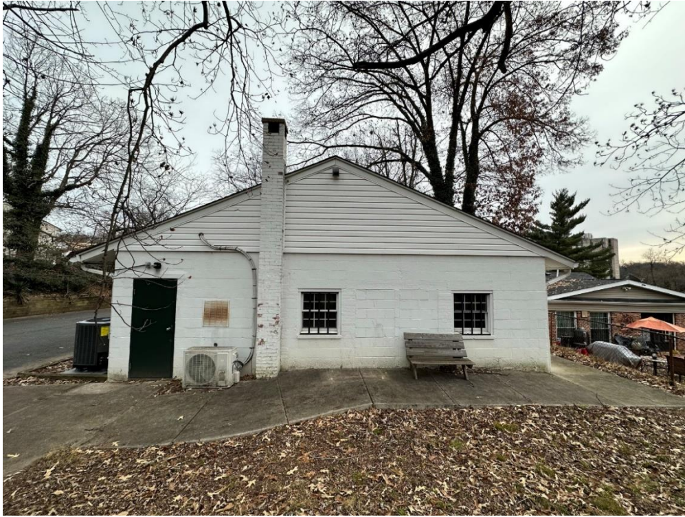
Figure 3: View of the west elevation.
