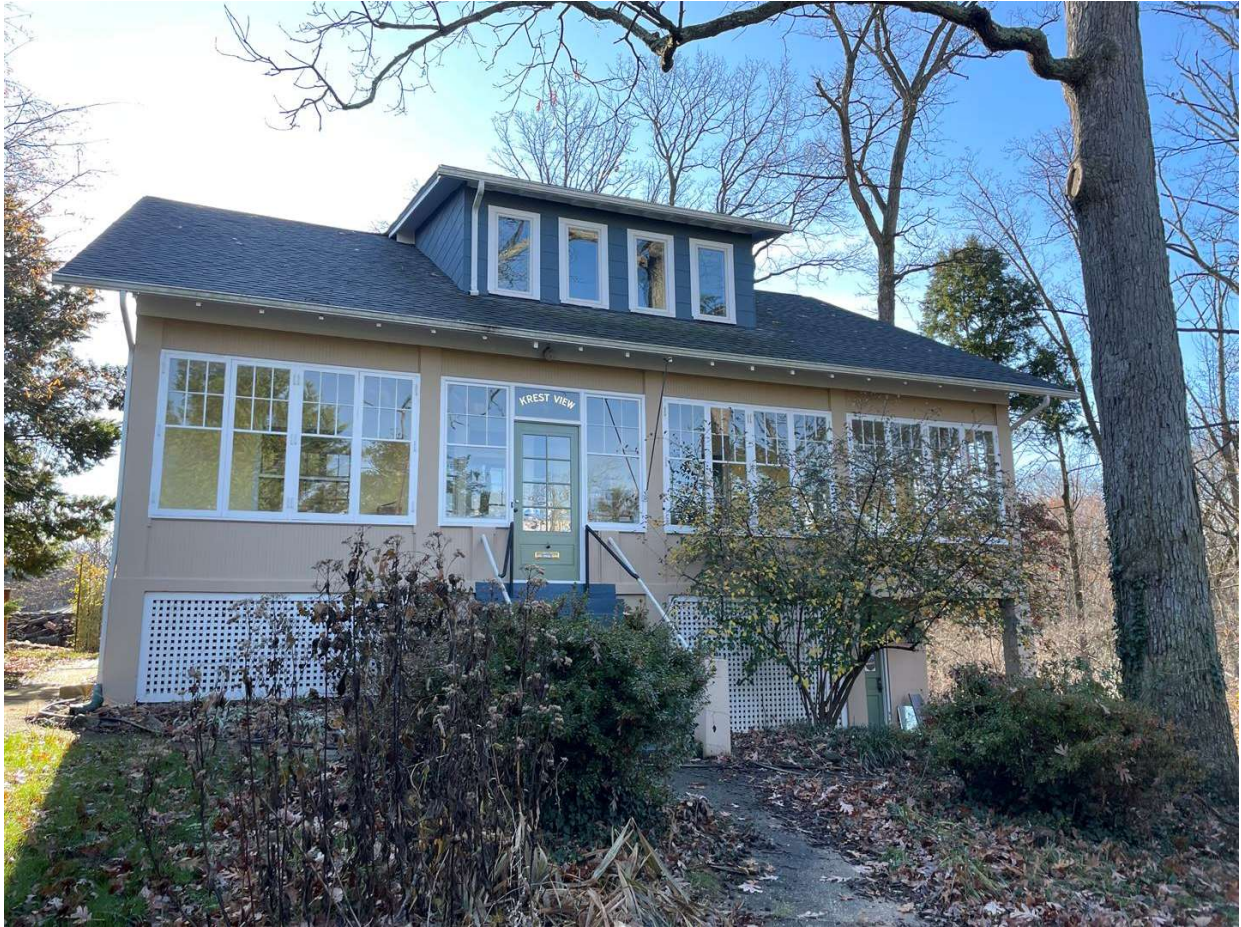
Figure 1: North (front) elevation of the Kress House, view to south, Nancy LiPira, December 9, 2022.
