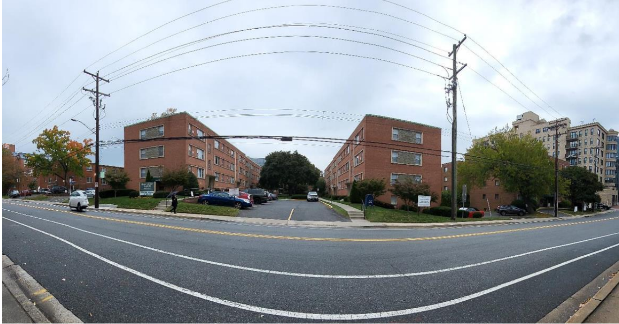
Figure 5 – Existing Conditions – Site’s Battery Lane Frontage
