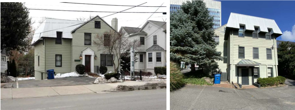
Figure 3: 4326 Montgomery Avenue, Front and Rear Views
