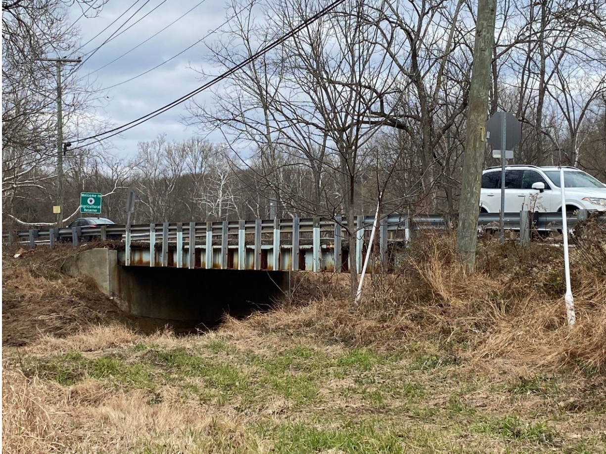
Figure 2: Brink Road Bridge over Great Seneca Creek – side view
