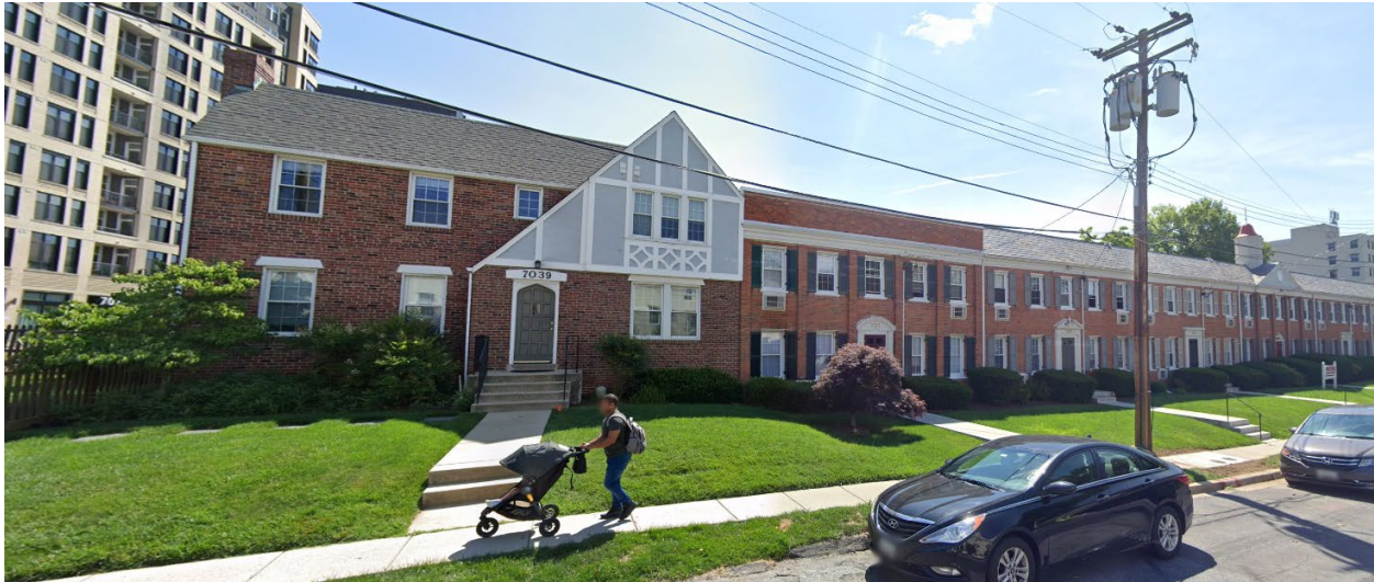
Figure 2 – View of Subject Property from Strathmore Street
