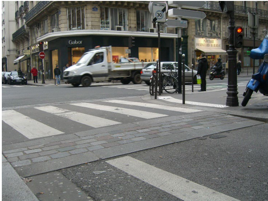
Figure 16: A raised crossing across a low speed, low volume street. Photo Credit: Vladimir Zlokazov
