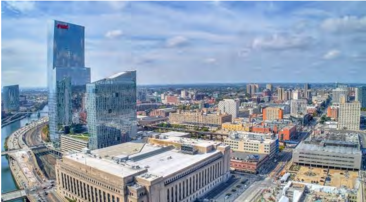
Figure 3.5: Aerial View of Part of University City District, Philadelphia
