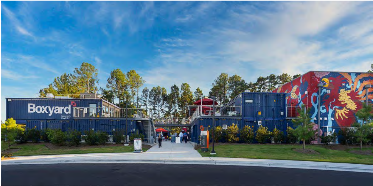
Figure 5.7: Boxyard RTP Outdoor Event Space
