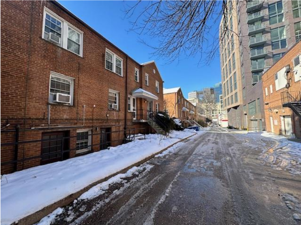
North View up alley Offutt Apartments to West side and Camille Apartments on East side
