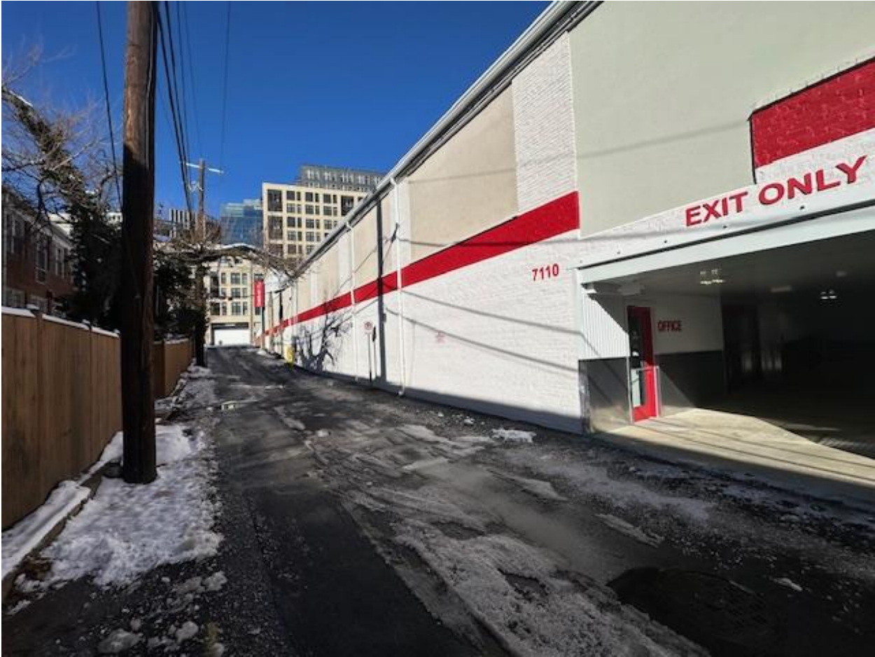
North View of Alley, 7025 Strathmore on West Side and Cube Smart Mini Storage on East Side
