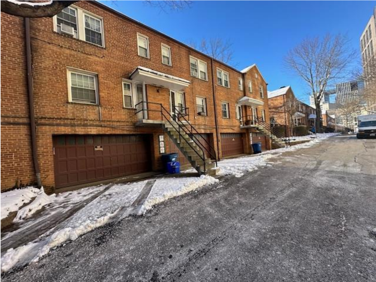
Offutt Apartments on west side of Alley
