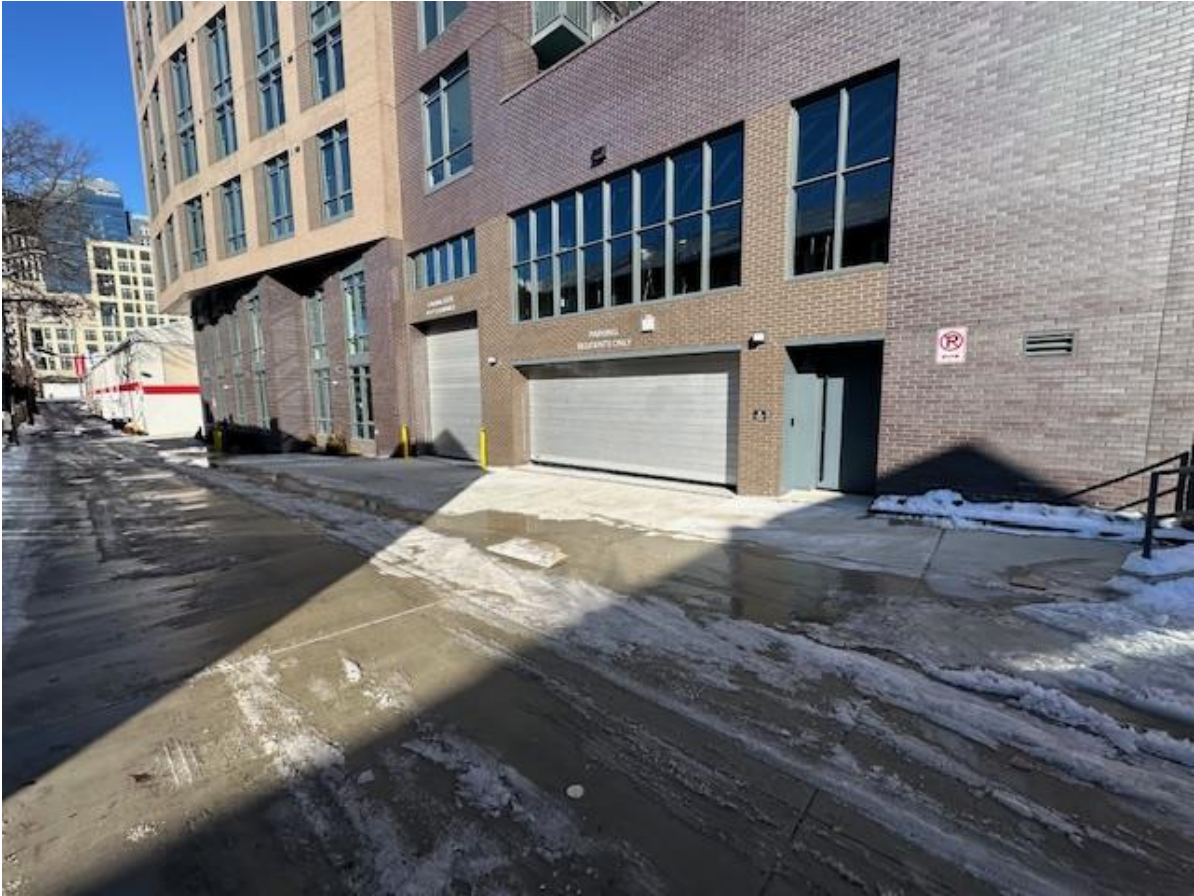
Camile Apartments Garage and Service Entrance of the alley
