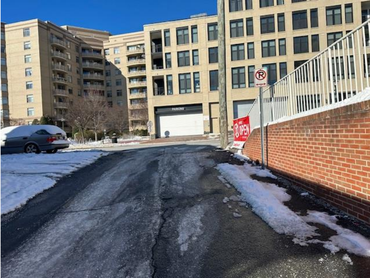
Alley Curb Cut from Woodmont Avenue, 7025 Strathmore on West side and Cube Smart Mini Storage on East side.
