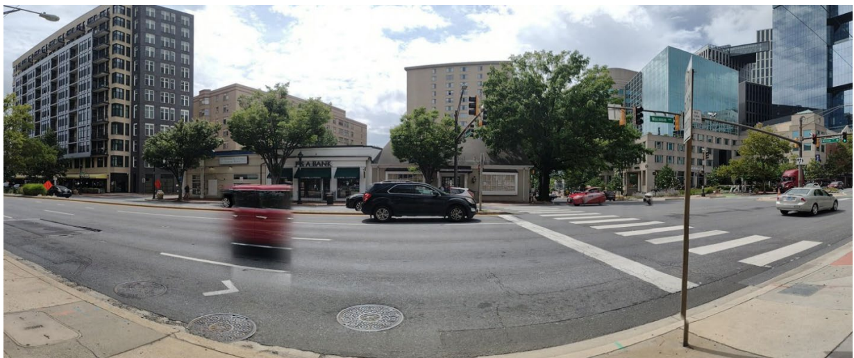
Figure 5 – Existing Conditions Images
