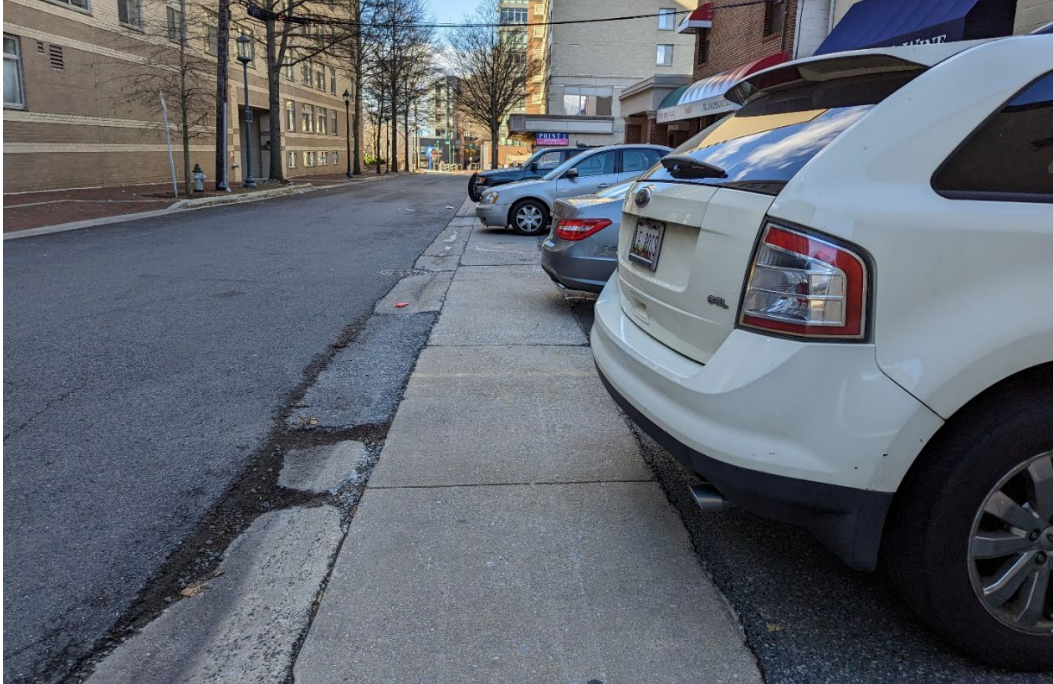
Figure 15 – Existing sidewalks on Miller Avenue
