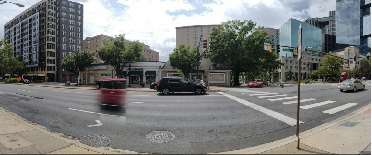
Figure 3 – Existing Conditions Images
