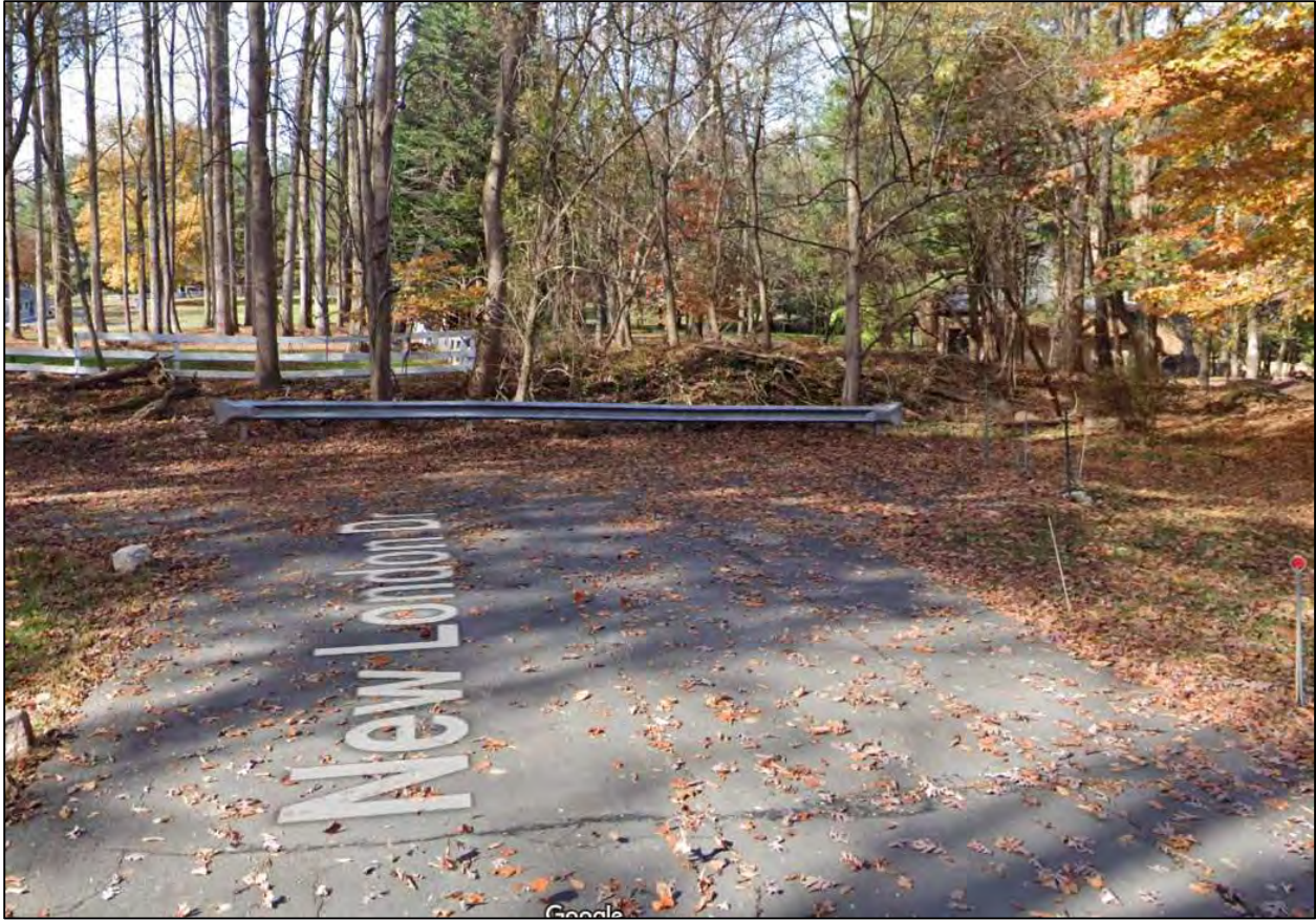
Figure 9 - Existing Non-Standard Temporary Terminus of New London Drive
