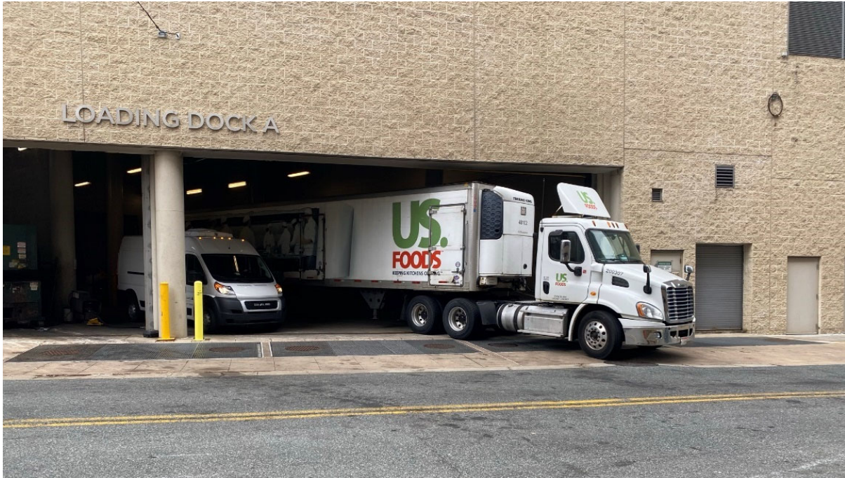
Figure X: Marketplace Lane loading dock with sidewalk blocked
