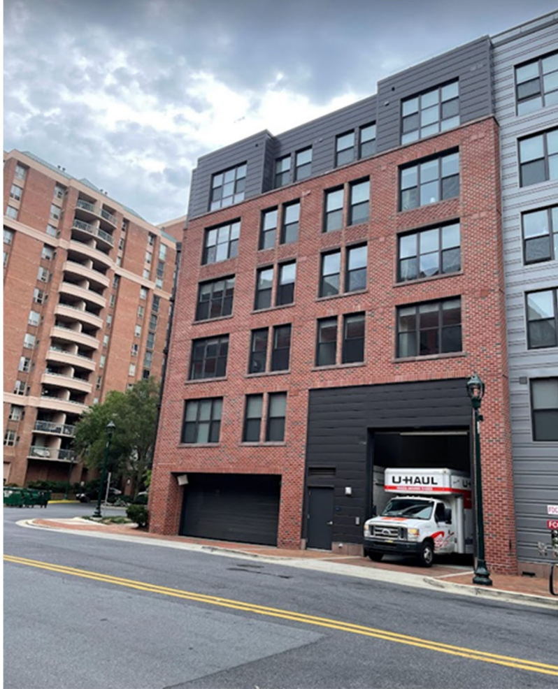
Figure 4: Internal loading for multi-family building showing truck impeding pedestrian area
