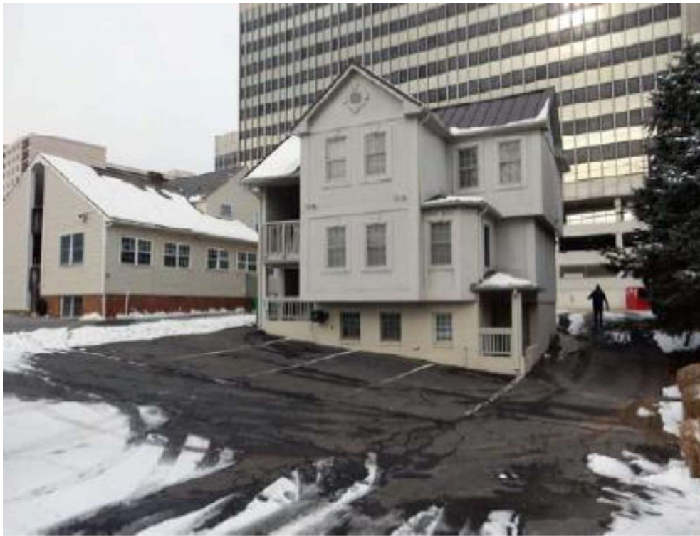
Figure 4: 4328 Montgomery Avenue, Rear View
