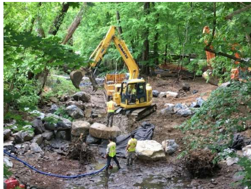
(still photo of Brashears Run stream "restoration" in Takoma Park, May 6, 2024)
