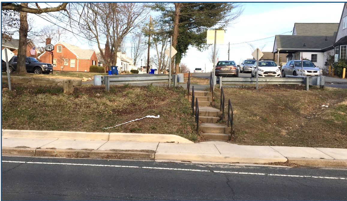
Figure 3: Stairway between North High Street and Morningwood Drive Looking East
