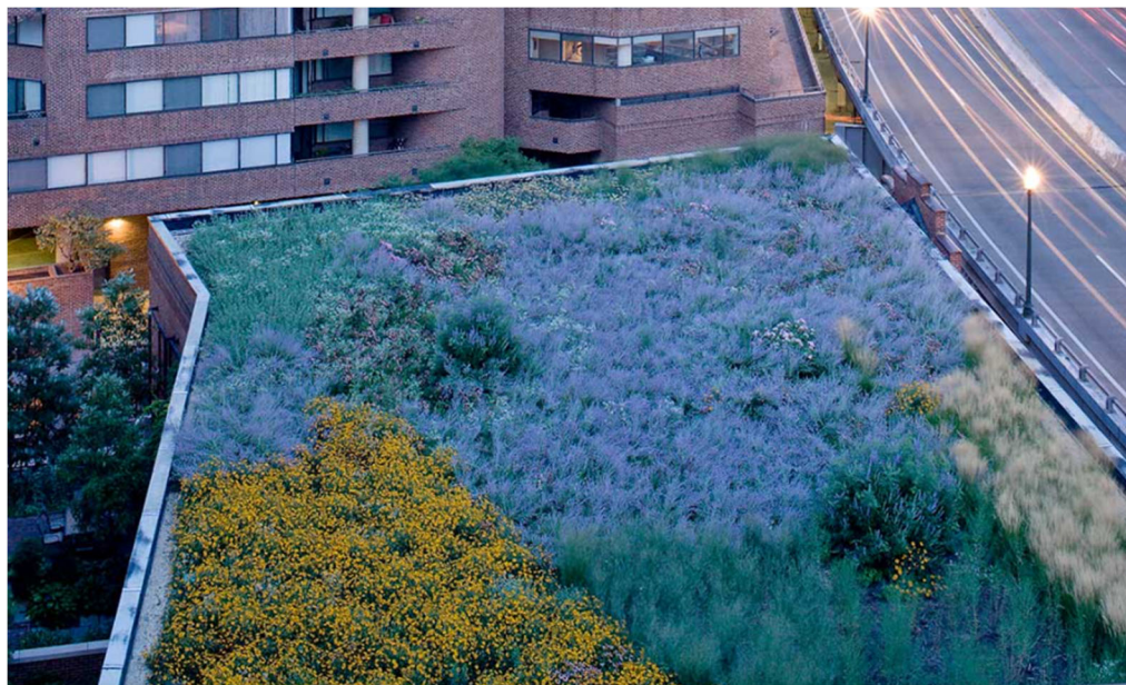
Case Study: Pepco Building in Georgetown 3303 water street – intensive green roof
