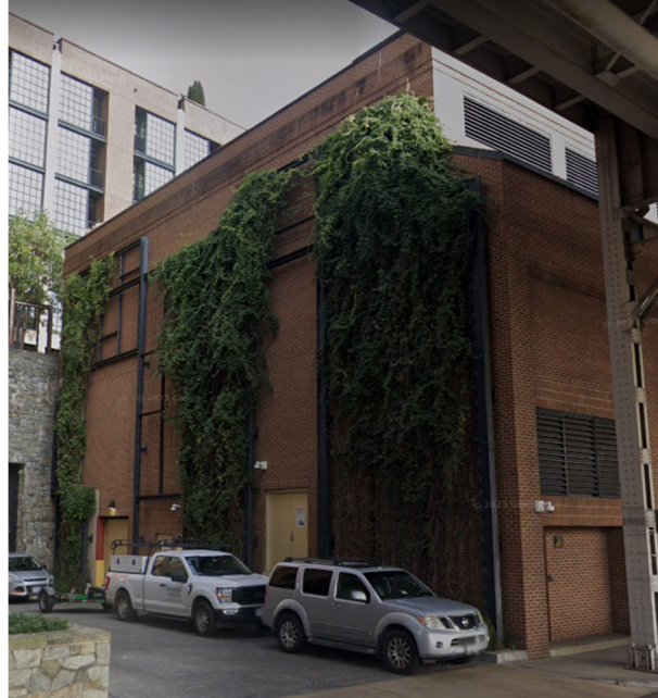
Case Study 2: PEPCO Substation in Washington, DC
