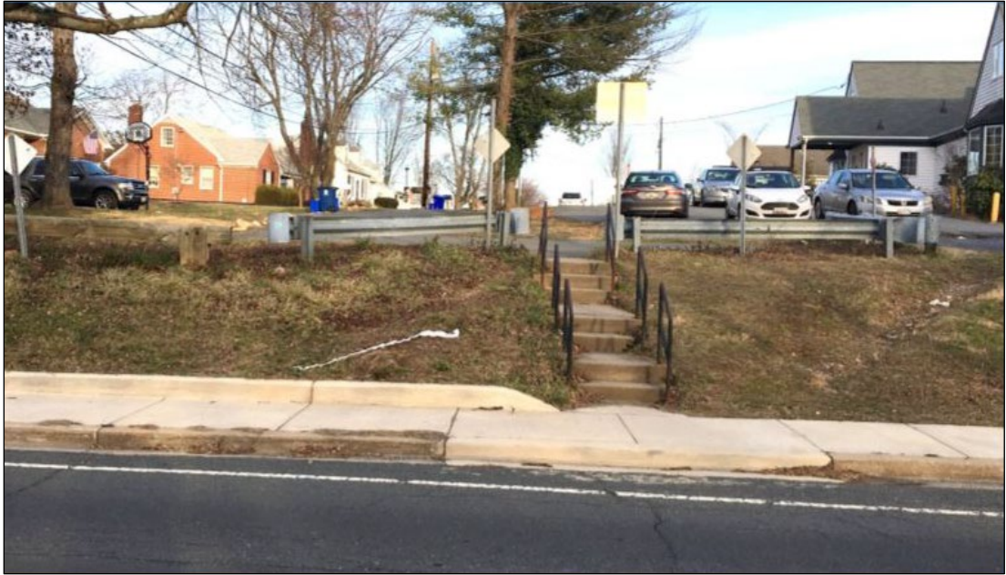
Figure 9: Stairway Connection to North High Street
