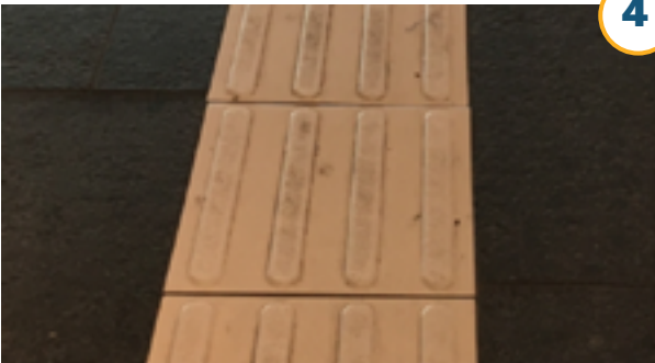
Figure 37. Example of tactile directional indicators
