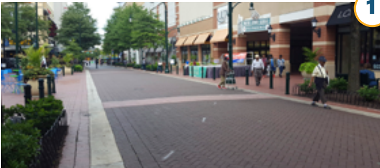
Figure 41. Example of a Valley Gutter on a Curbless Street
