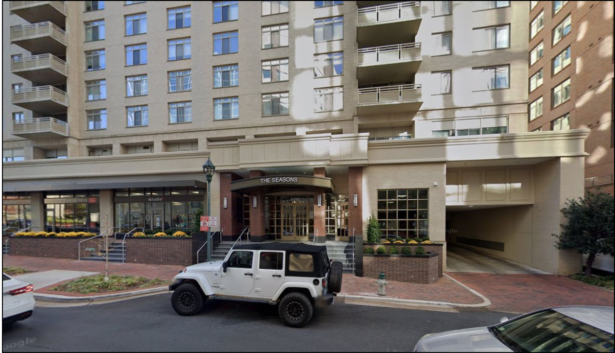
Figure 3 – Subject Property from Bethesda Avenue looking south
