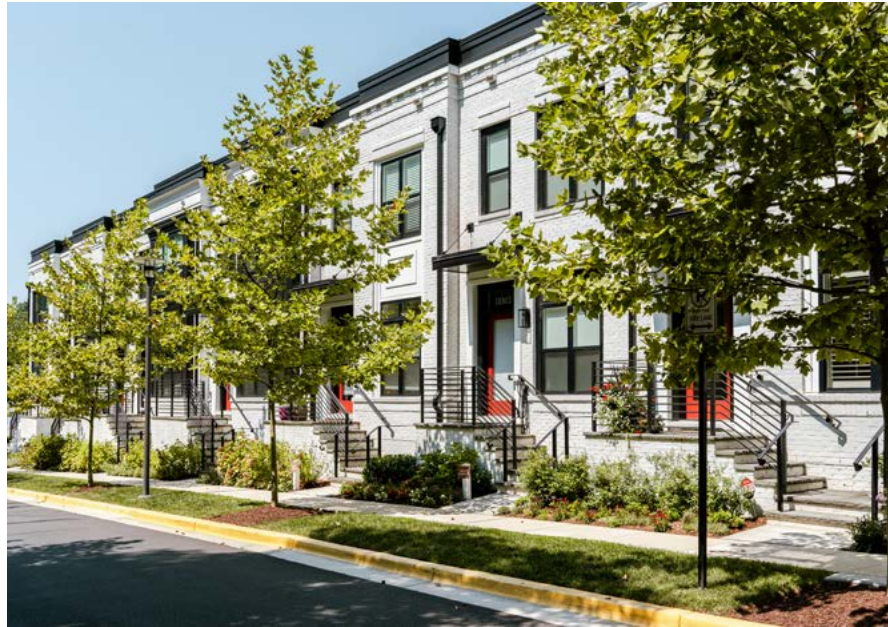
Figure 17: Townhouses in Cabin John Village
