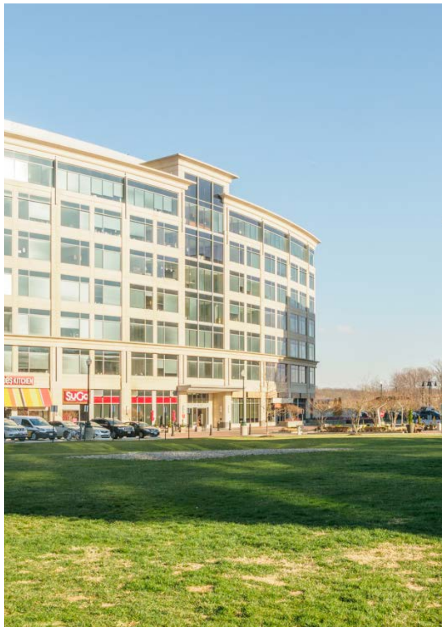
Figure 42: Office buildings with open space on east side of Park Potomac
