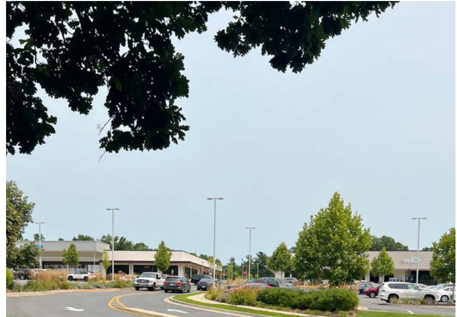
Figure 18: Roadways within Cabin John Village
