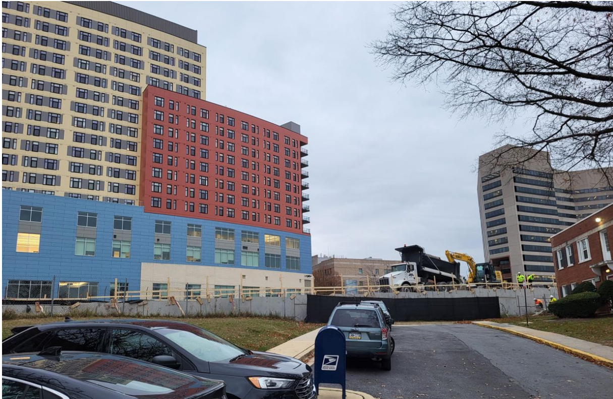
Figure 4 – Purple Line Construction at Falkland North December 4, 2024
