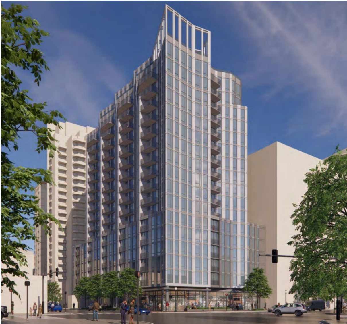
Figure 4 – Rendering of proposed Site Plan looking southeast towards St Elmo/Old Georgetown Road
