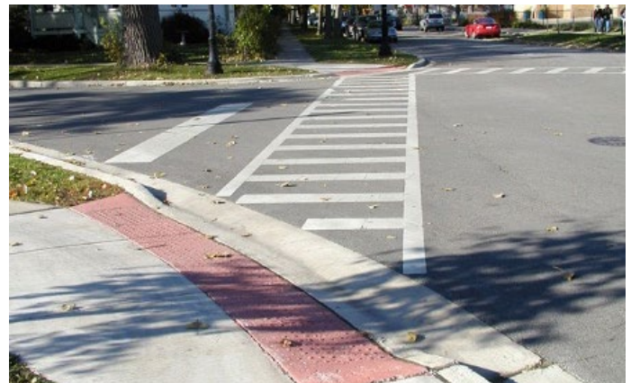
Figure 37: Example of curb ramp that is not aligned with crosswalk.
