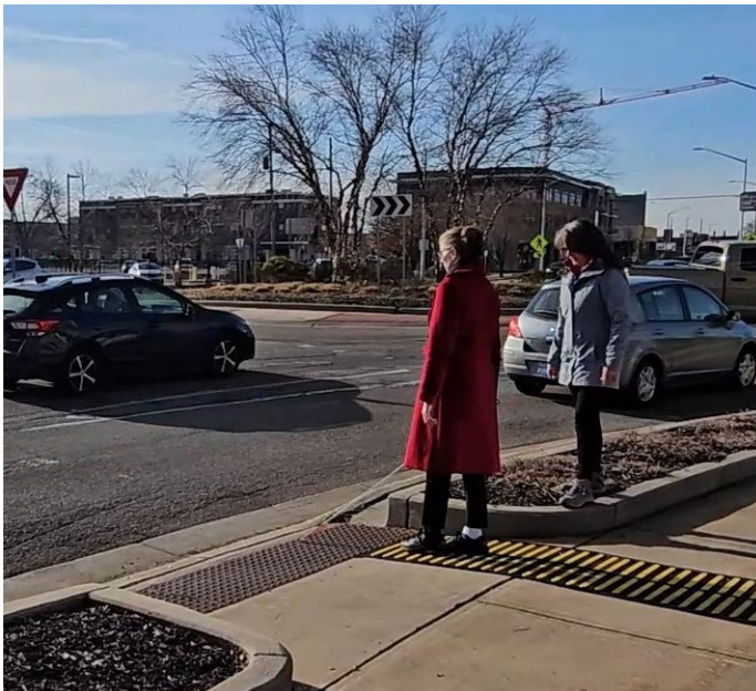
Figure 13: Example of sidewalk alert TDI (Source: Jennifer Graham, Accessible Design for the Blind)
