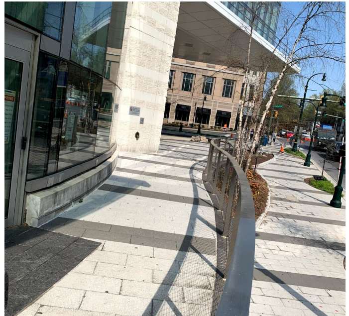
Figure 19: The walkway outside Brigadier General Charles E. McGee Library in Silver Spring features alternating bands of dark and light pavers which may look like steps to a person with low vision.
