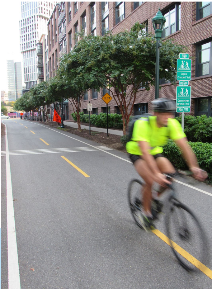
Figure 22: Path with edge lines
