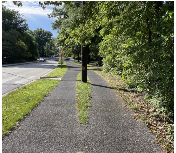
Figure 21: A shared use path splits around a utility pole. The wedge of grass provided is a non-prepared surface that may help people with vision disabilities navigate around the obstacle. Retroreflective edge lines could also be used to help define the correct path in this context.
