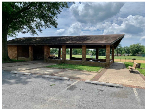
Wheaton Forest Local Park Picnic Shelter
