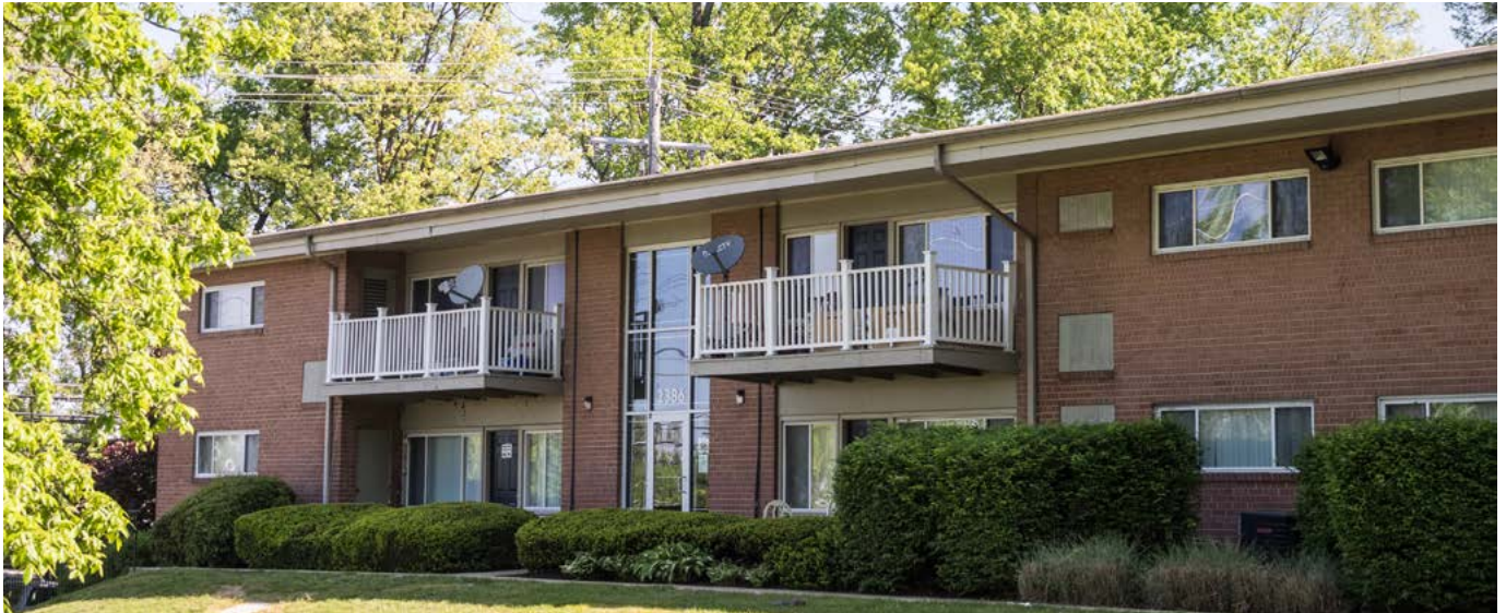
Figure 13: This photograph shows the Glenmont Forest apartments.
