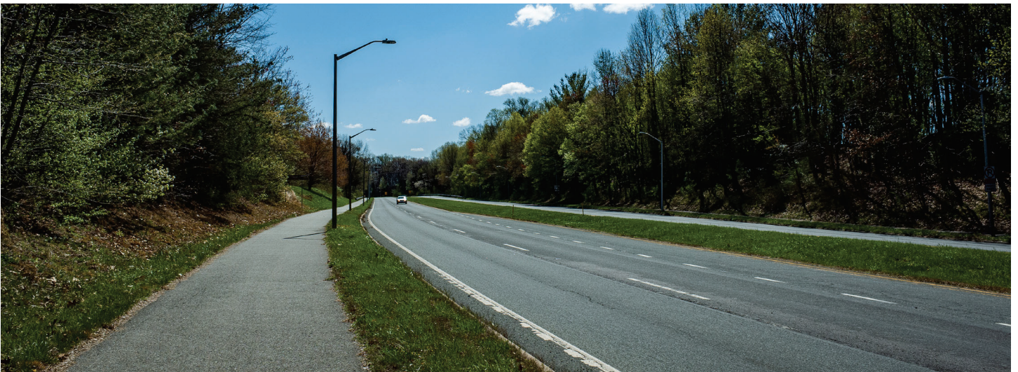
Figure 2-100. Great Seneca Highway from Longdraft Road to Mateny Road
