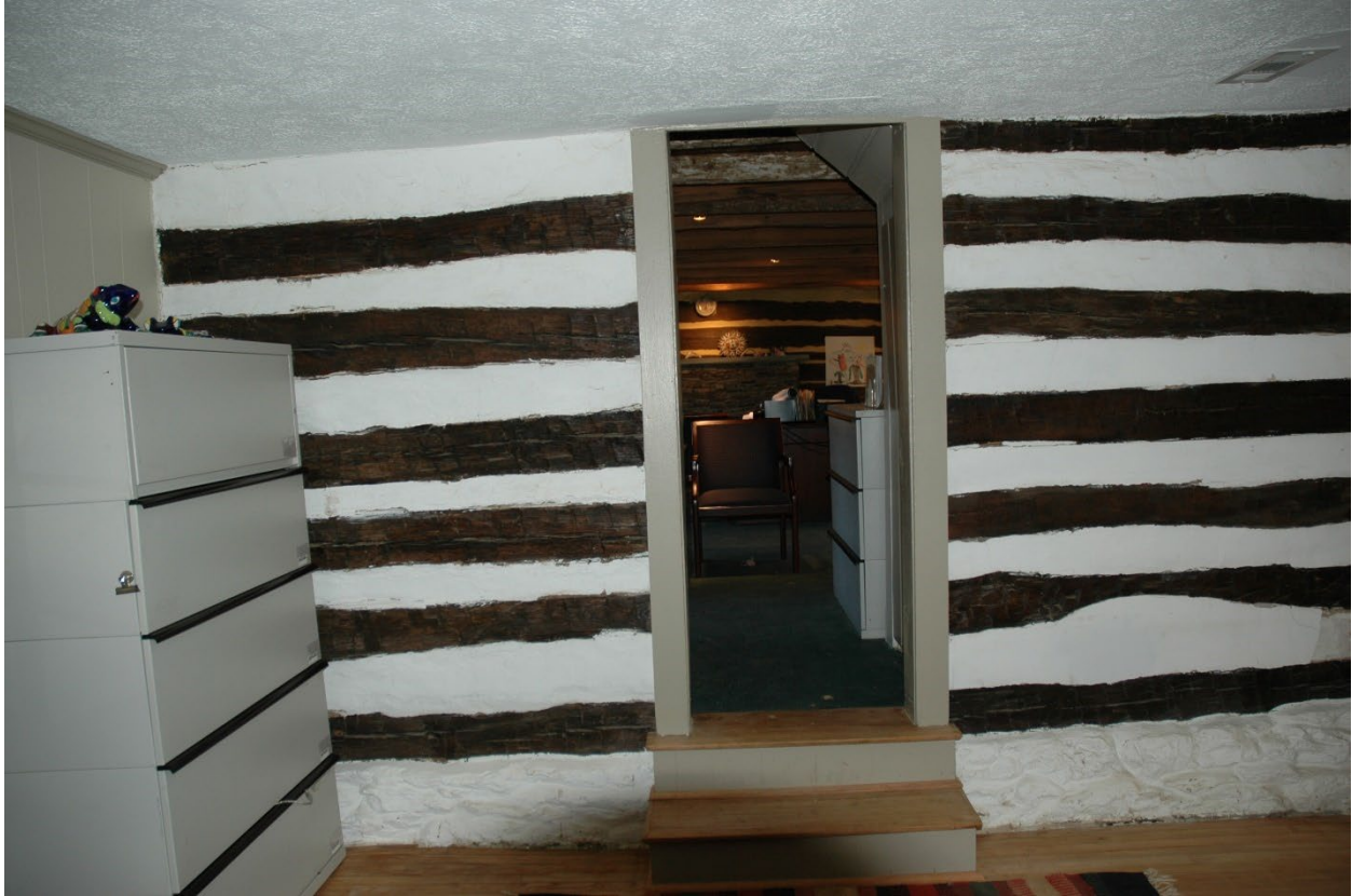
Figure 12: View of the interior of the Wilson H. Cecil House, 2008. The opening is in the north elevation of the log house obscured by the later addition. Source: Montgomery Planning.
