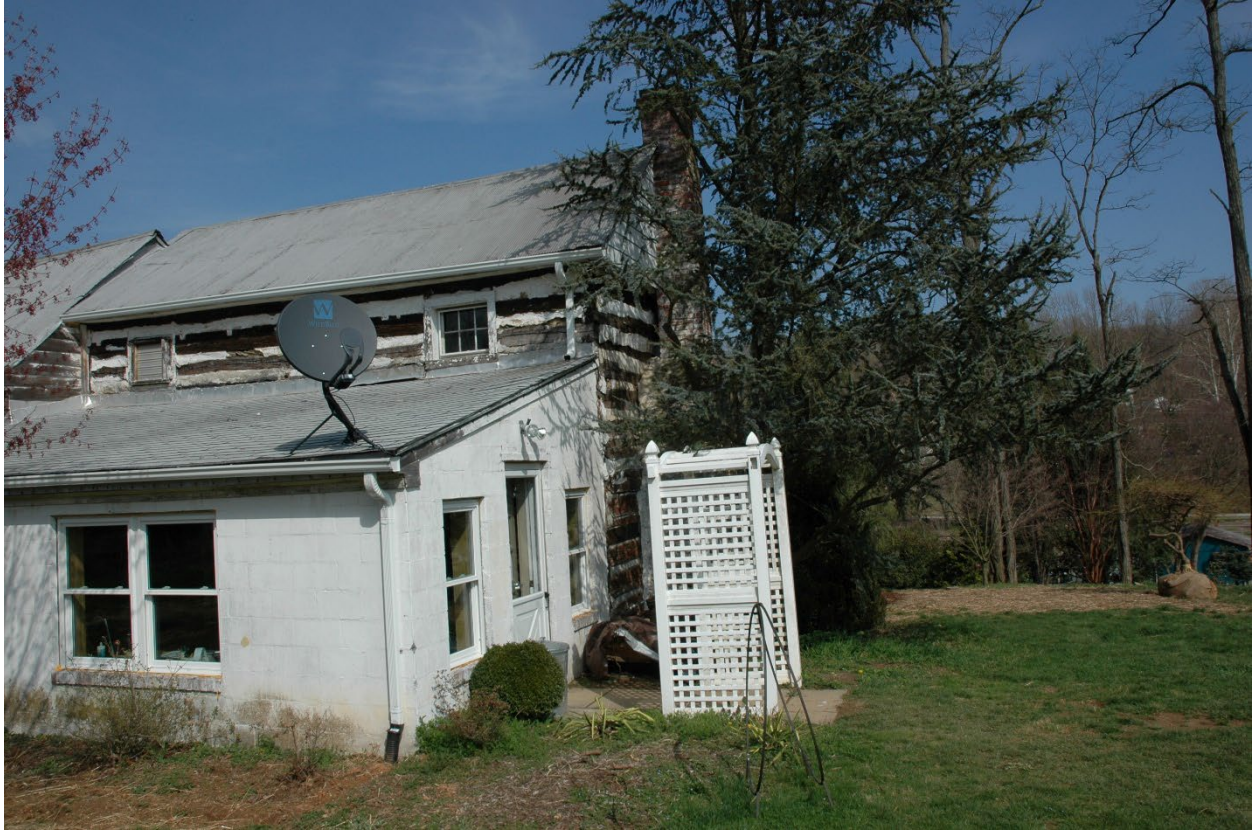
Figure 10: View of the south and west (rear) elevations of the Wilson H. Cecil House, 2008. Source: Montgomery Planning.
