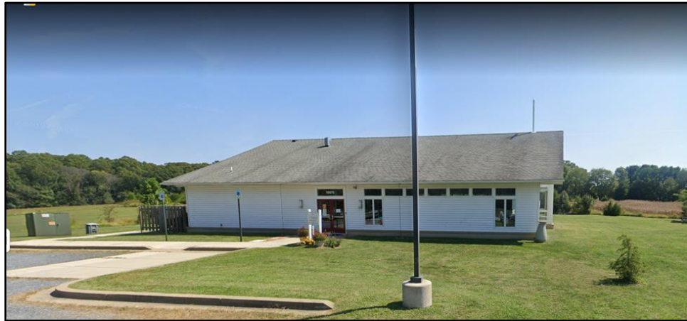
Figure 4 – Existing Church Building
