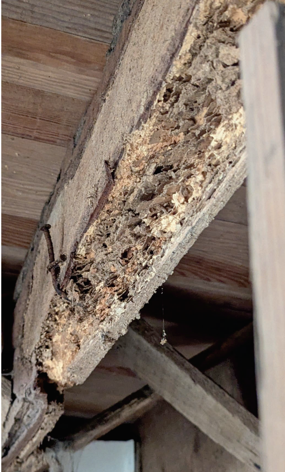
Figure 30: Damage to joists under house, Montgomery Planning, 2025.
