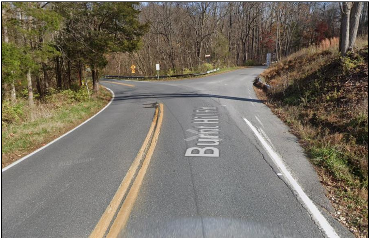
Figure 5: Burnt Mill Road at Kingstead Road, Looking North
