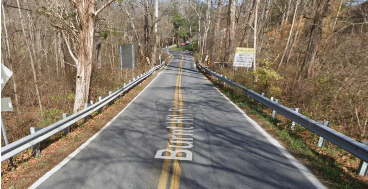
Figure 6: Burnt Mill Road at Existing Bridge, Looking North
