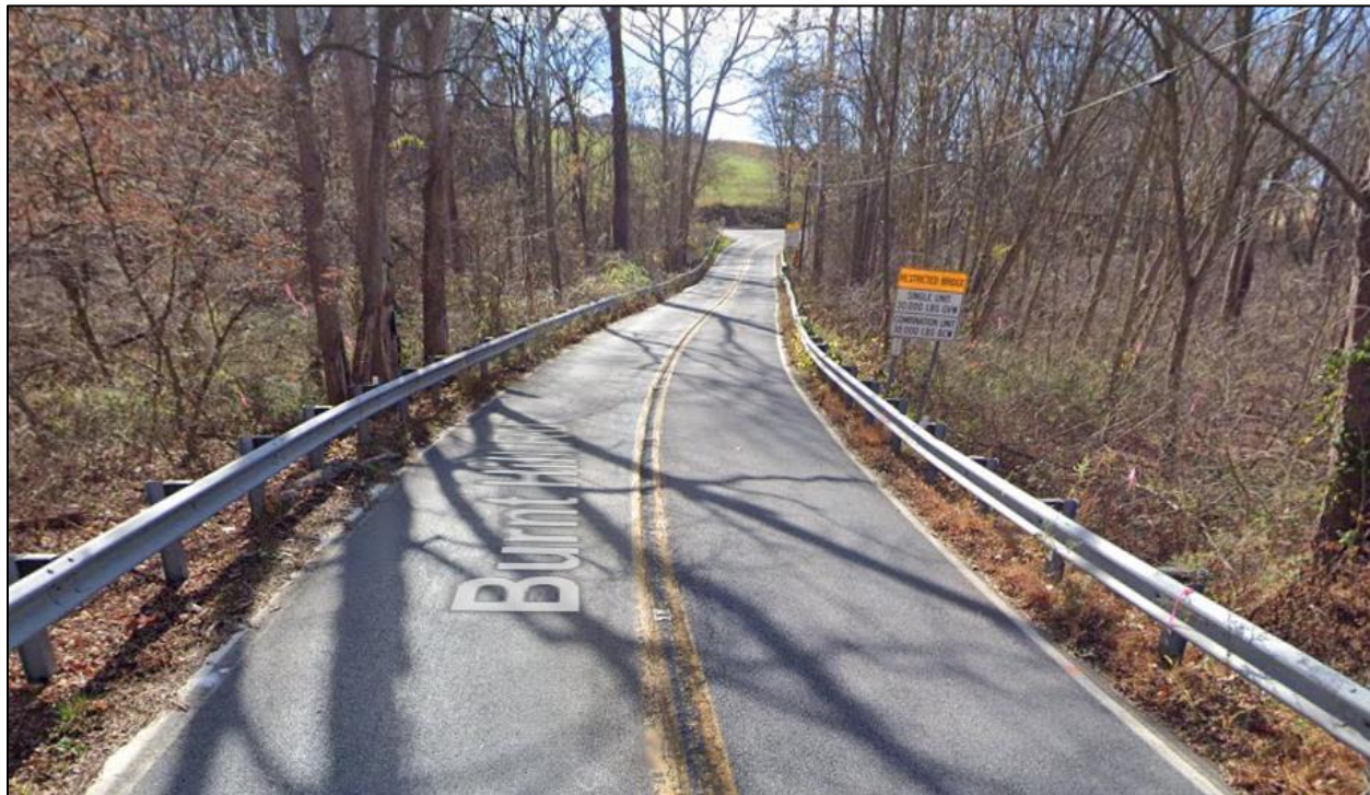
Figure 7: Burnt Hill Road at Existing Bridge, Looking South
