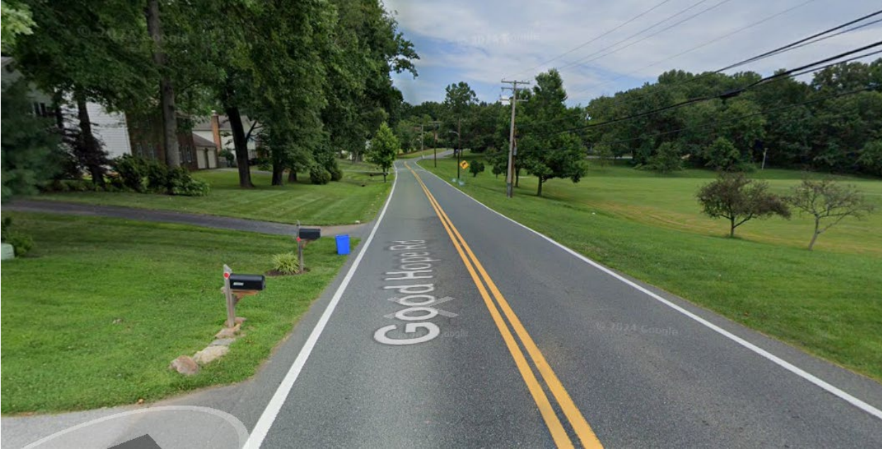
Figure 6: Good Hope Road Between Rainbow Drive and Spencerville Local Park, Looking North
