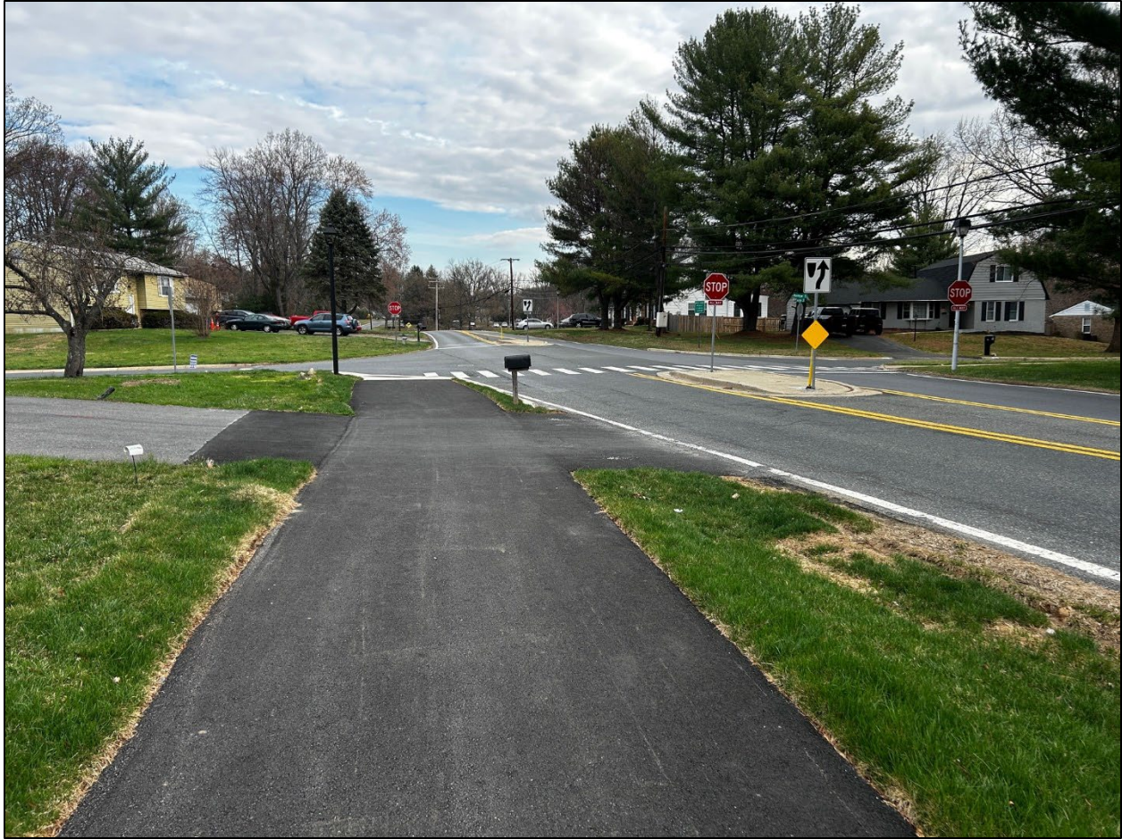
Figure 2: Existing Good Hope Road Sidepath Terminus at Rainbow Drive, Looking North
